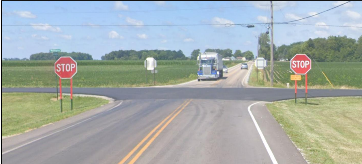
Figure 3 – Intersection Conditions (on east leg looking west)
