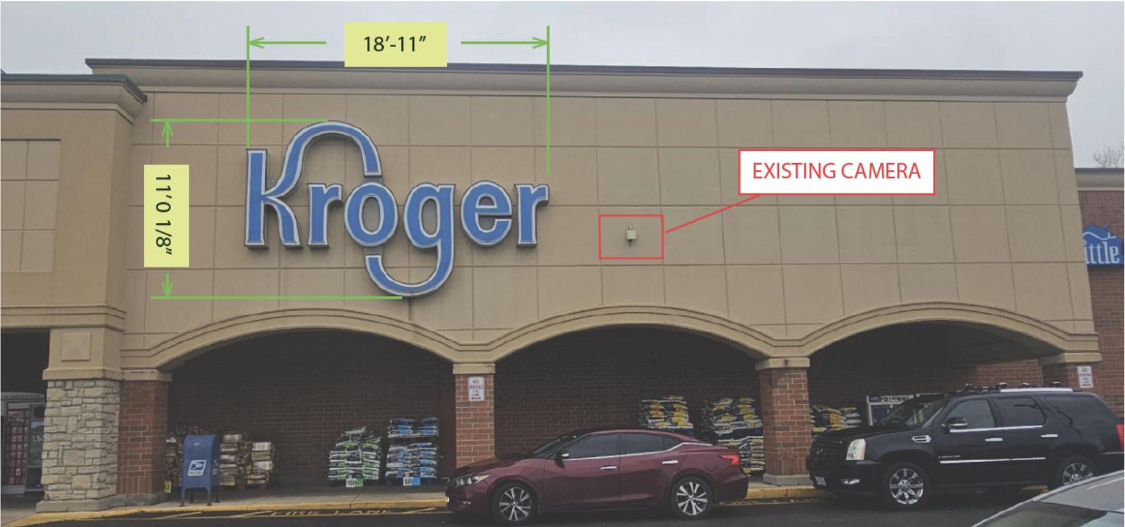
EXISTING SCOPE OF WORK: FRONT ELEVATION - REMOVE THE CURRENT BLUE KROGER LETTERS AND GO BACK WITH NEW BLUE SET OF KROGER LETTERS AND CART CURRENT SET OF LETTERS ARE 11'1/8" H X 18'11"W. INSTALL NEW OHLQ LETTER SET.
