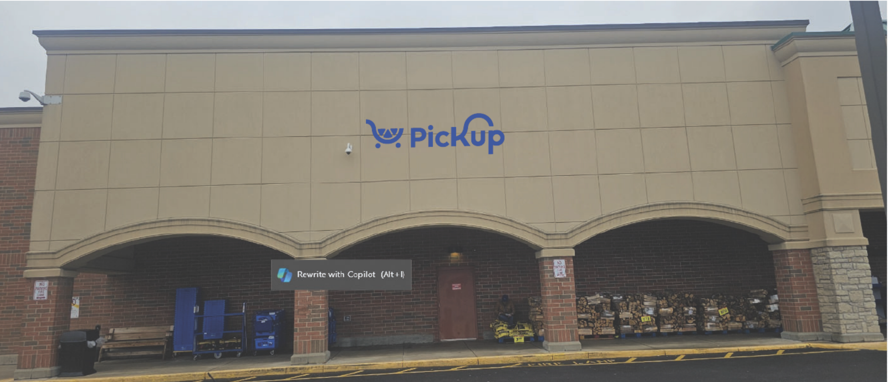
EXISTING SCOPE OF WORK: FRONT ELEVATION - REMOVE THE LIQUOR SIGNAGE AND GO BACK WITH 24" BLUE PICKUP LETTER SET-CURRENT SET OF LETTERS ARE 23-1/2 HIGH AND SPAN 8-8-1/4" THE WALL AREA THAT SIGN GOES ON IS 14'5/8" H X 63-1-3/4".
